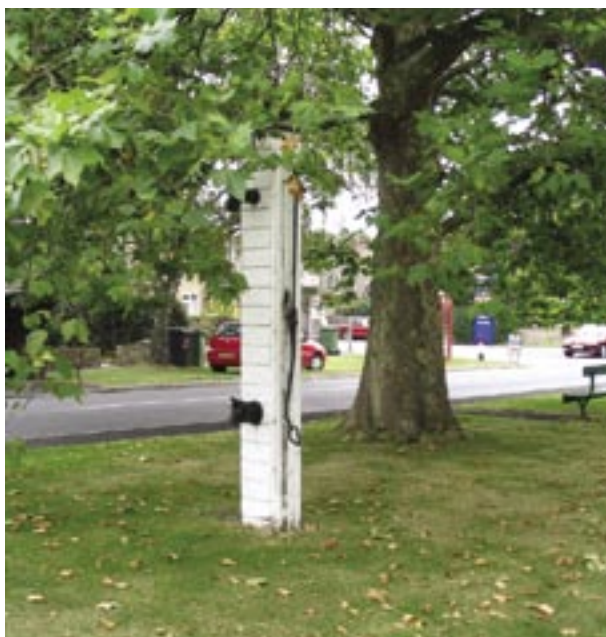
Grade II Listed water pump
